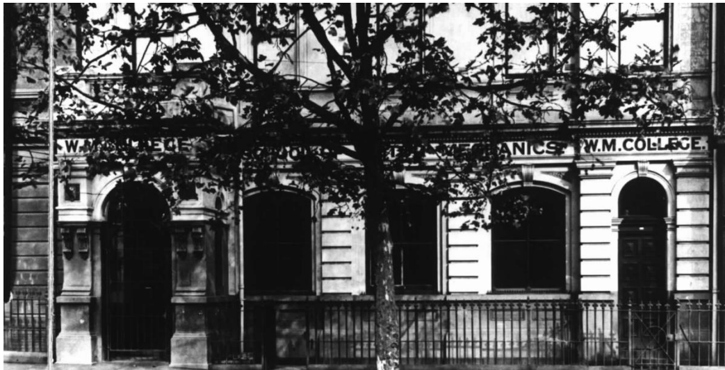
Image 28 RMIT University Photographer, SN Rodda School of Motor Mechanics building. 1940. Image No. 1934. PH2.4.9. RMIT University Archives, Melbourne.
