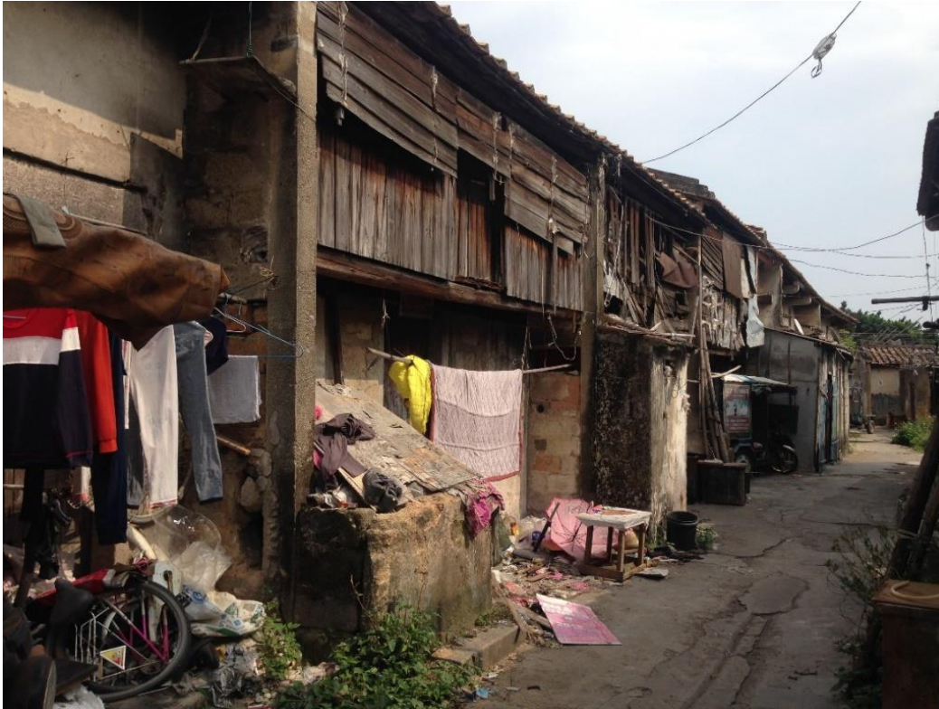
Figure 8 Appearance of one laozhai from the inside. 6
