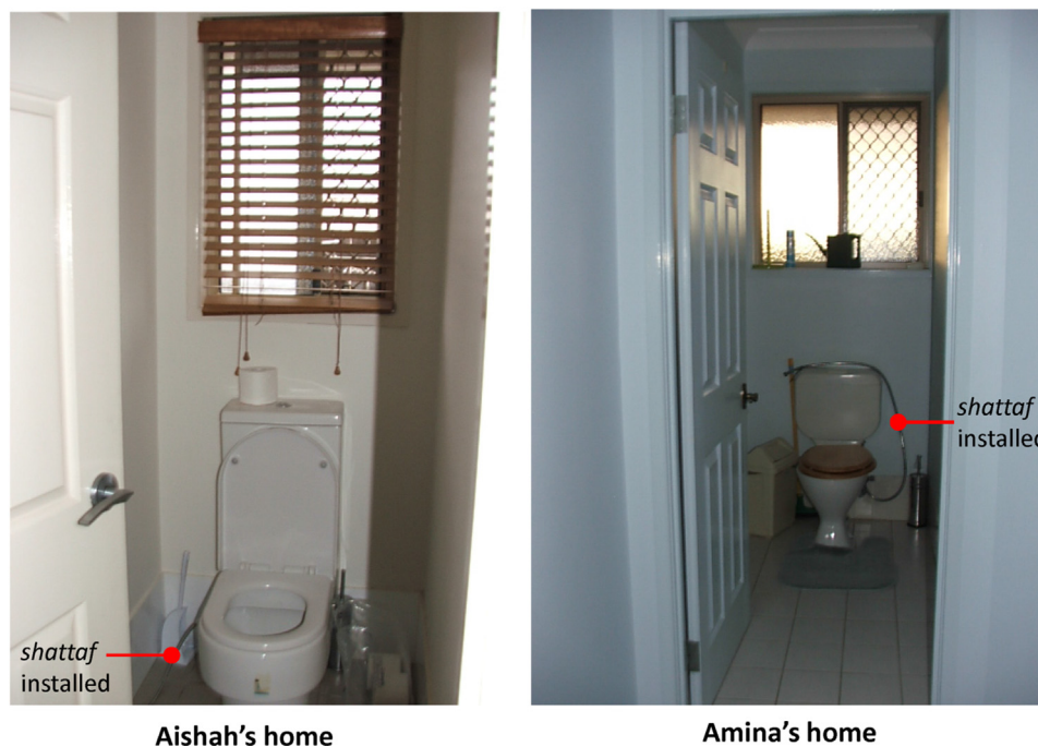
Fig. 3 Installation of shattafs in Aishah's and Amina's homes. Source: Author.
