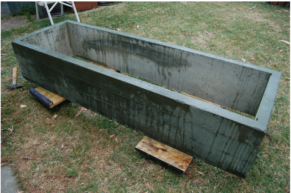
Figures 34 and 35. Formwork with poured cement, July 2006; Cast form (plinth) revealed after formwork taken away. July 2006.
