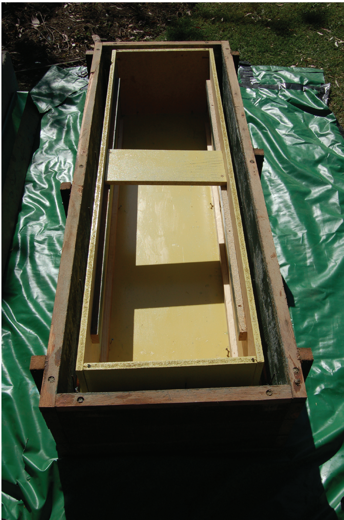
Figure 33. Formwork or mold for casting plinth, July 2006.
