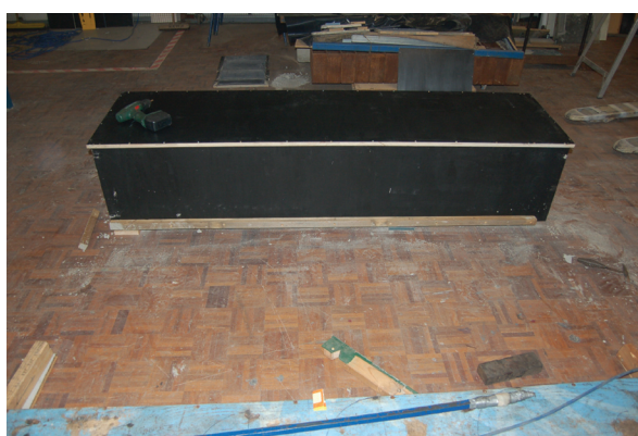
Figures 67 and 68. Form-ply casing; the new work as revealed after casting, 2007.
