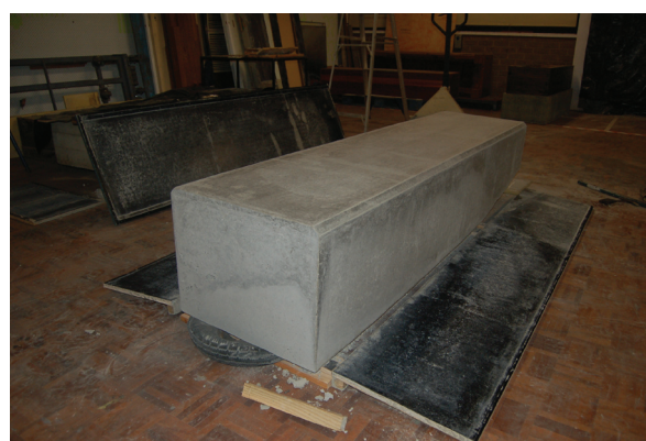
Figures 67 and 68. Form-ply casing; the new work as revealed after casting, 2007.
